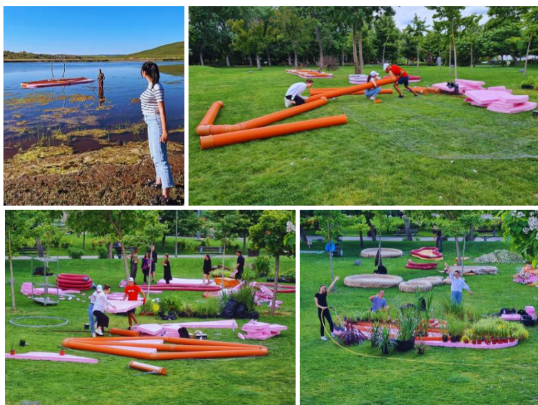
Fig. 3. Construction sequence: (upper left) practical buoyancy and stability check on water; (upper right and bottom) on-site assembly and planting during implementation
